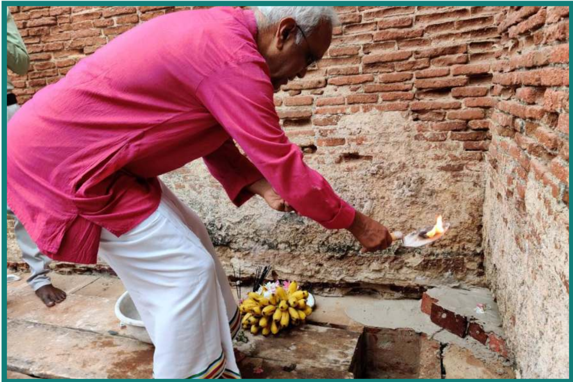
The Pooja was performed on 06-Dec-2019 to mark the deposition of the Lime-Mortar brick concrete
