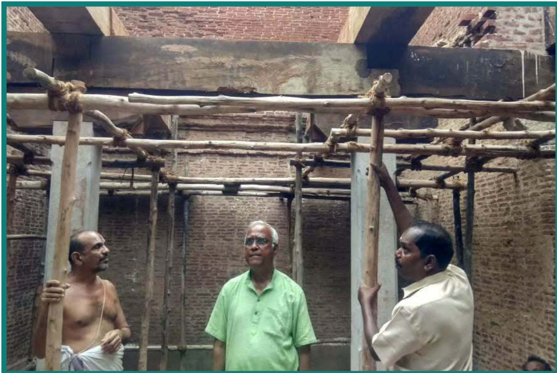
Granite stone columns were positioned in place.
