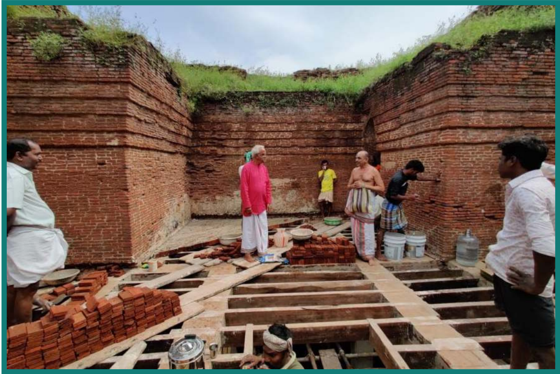
The Lime-Mortar cum special bricks are being placed in position on Dec 2019
